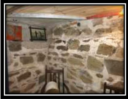
Figure 18. Basalt used to form the foundations and walls of the cellar in an historic inn at Bathurst.
