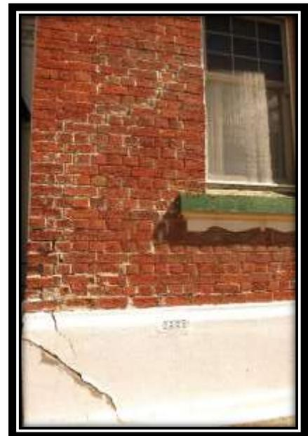
*Figure 14. Cracking brickwork and rising damp is common in many older buildings on the old alluvial flood terraces.*
