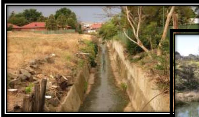
*Figure 12. The chanelised, straightened and deepened course of today's Jordon Creek. Note the broad flat form of the original floodplain to the side of the drain.*
