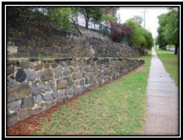
*Figure 17. Wahluu/Mt Panorama basalt, originally used to form street guttering in old Bathurst has been reused to form retaining walls at Bathurst High School.*
